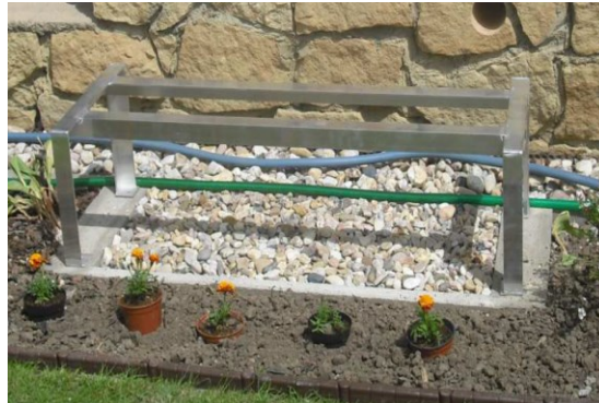
Image 10: Example of a heat pump base design
